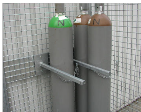
Fixture with safety chain
